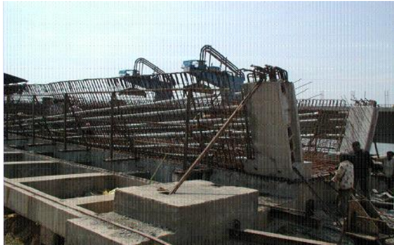
Fig.2.2.internal prestressing of a box girder (courtesy: cochin trust ,kerala)
