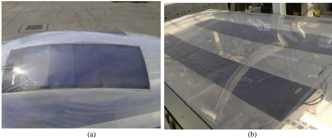
Fig. 9 Typical ETFE cushions integrated photovoltaic/thermal systems. (a) Two-layer ETFE cushions with photovoltaic integrated on top layer. (b) Three-layer ETFE cushions with photovoltaic integrated on middle layer [31].
