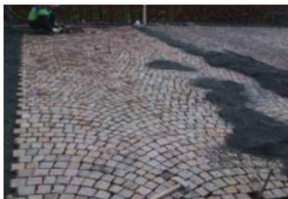
Figure 11. Solutions to use permeable pavement
